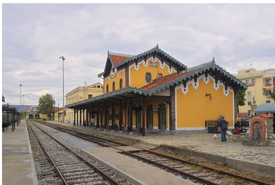
Figs. 7 and 8: Volos train station. Above front of the building and 600 mm track to Milies (ca. 1910), below the station today with platform for direction Velestino and Larissa. 14
